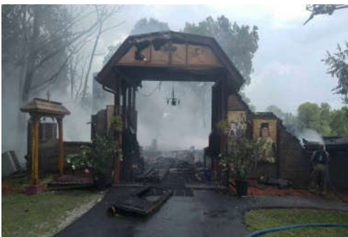
The damage to the church was extensive.
